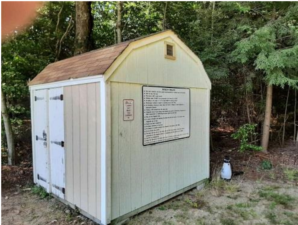
The shed at the Nottingham Town Beach after Wednesday afternoon, July 20, 2022.
