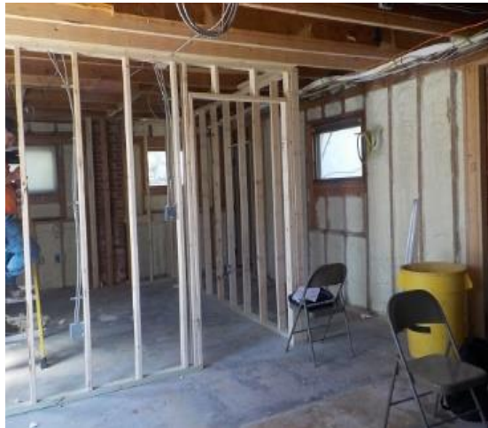
The Nottingham SA's offices are taking shape
