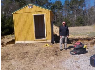
Carl Edin supervising the conduit connections at Marston
