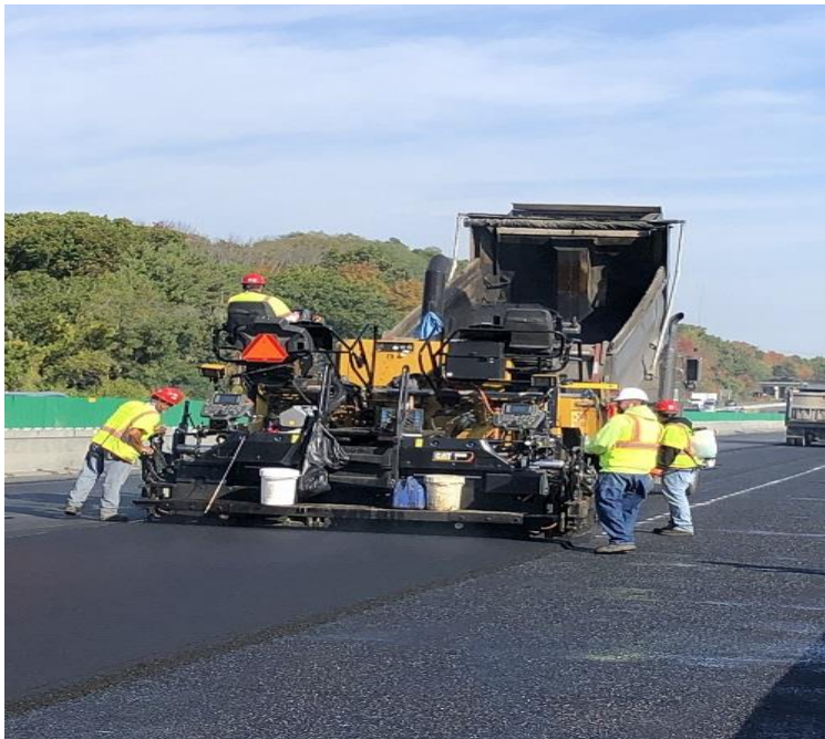
Brox repaving a road Photograph by Brox Industries
