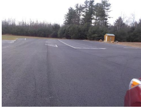
Marston paved and parking lines painted.
