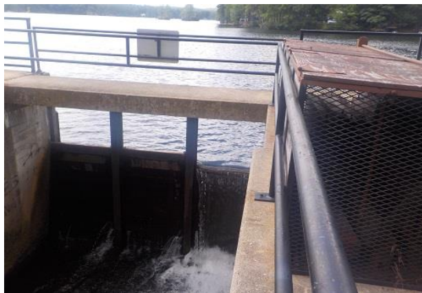
Dolloff Dam from the back side with 2 stop logs pulled.
