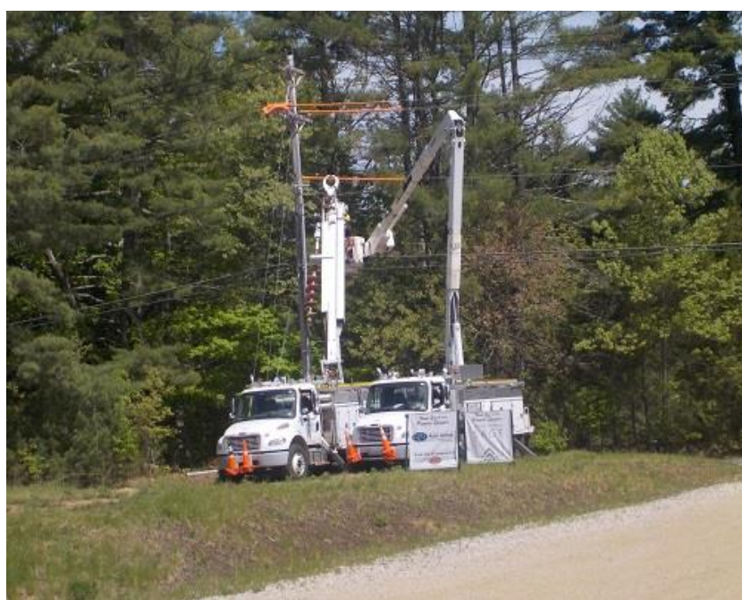
New Hampshire Electric Co-op crew connecting Marston to the powerlines
